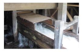
To direct the flow of water a sluice would carry the water from the pond or river to the water wheel or water turbine and then away from the mill once it passed through the water wheel or turbine.
