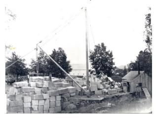
Originally powered by horses, a very real innovation was the arrival of a 12hp steam engine to power the derrick. This was eventually replaced by a 20hp steam engine.
