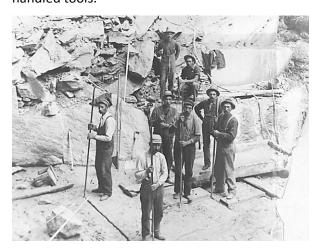
The quarry operation required that they dig down ever deeper into the stone for new blocks. While gravity was a friend in this downward process, it quickly became foe when it was time to lift the blocks to the surface. The cut blocks were generally 3'x6' or 5'x7' weighing hundreds of pounds. The quarry eventually reached a depth of 134' (the equivalent of a 14-story building only down, not up). Only a derrick allowed them to reach this depth.
