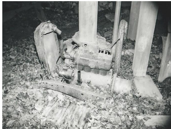
THE REMAINS OF THE GASOLINE ENGINE BROUGHT INTO THE MILL TO REPLACE THE FORMER WATER WHEEL
