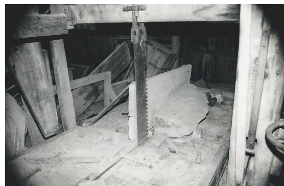
UP AND DOWN SAW IN MILL AS IT WAS WHEN MILL CLOSED WITH A PARTIALLY CUT STONE STILL ON THE SAW TABLE
