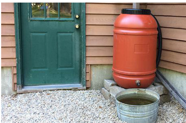
Above: Rain barrel to catch rainwater runoff from roof Source: NH Department of Environmental Services
