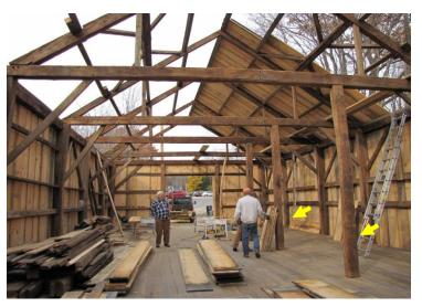
The trees cut from the town forest had by now been sawn into planks for the siding and roof. The wooden uprights that appear to be not in keeping with the symmetry of the timber frame ultimately would become a part of the small loft area which was original to the old barn. Windows would be cut into the siding to match those in the original structure. A metal roof cover would also be applied.
