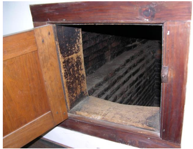
SMALL DOOR IN WALL OF ROOM AT SIDE OF FIREPLACE
