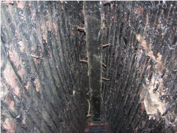
HOOKS ALONG THE ROOF OF THE CHAMBER
