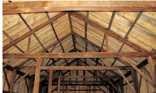
THE MUSEUM BUILDING UNDER CONSTRUCTION
